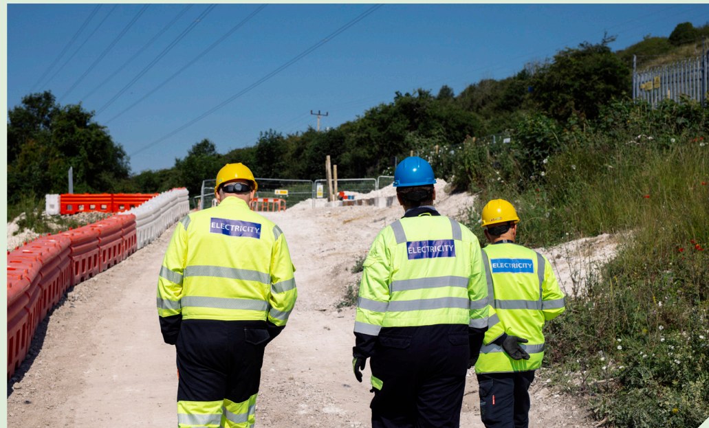
Caption: Construction underway on Fort Widley 132kV cable replacement project
