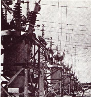
AEI SWITCHGEAR - TYPE BL BUSHINGS
