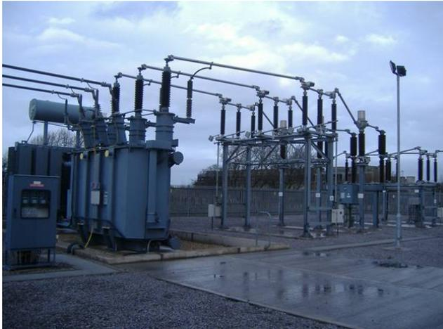
132kV Grid Substation showing main power conductors at high level but control circuits located in cubicles at lower level
