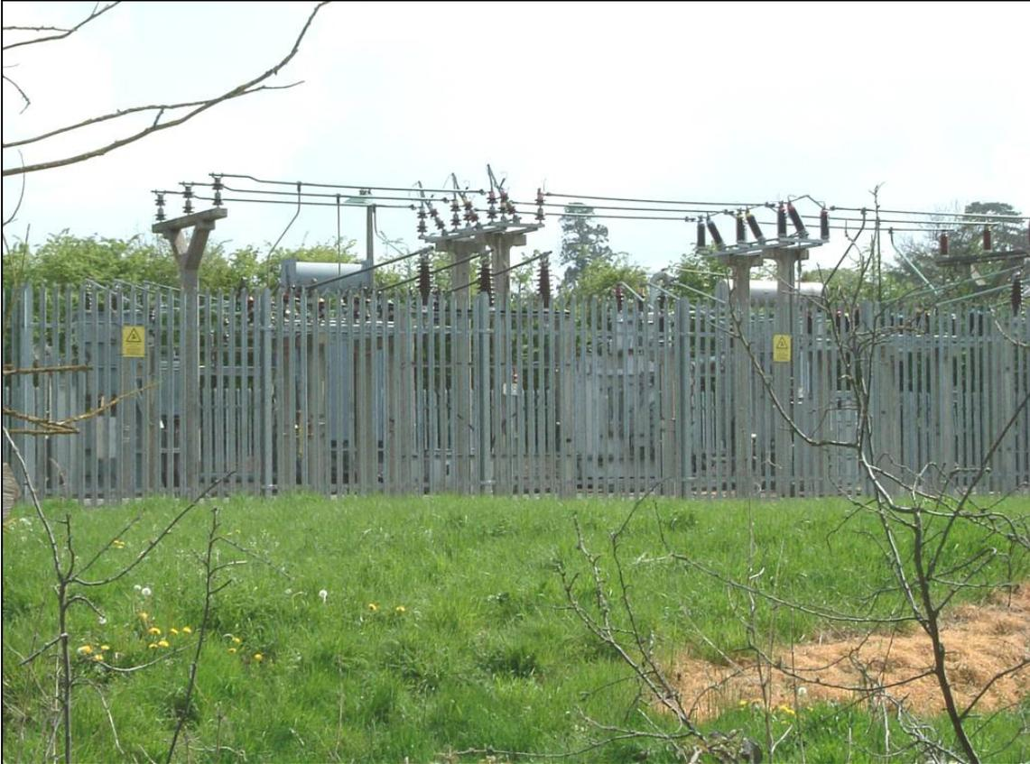
**Photograph 6 - Primary Substation showing equipment operating at 33kV and 11kV**
