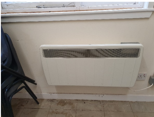
Figure 24 A typical electrically heated convactor unit found in substation buildings.
